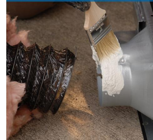
5. Connect the flex duct at both ends using flex duct ties.
