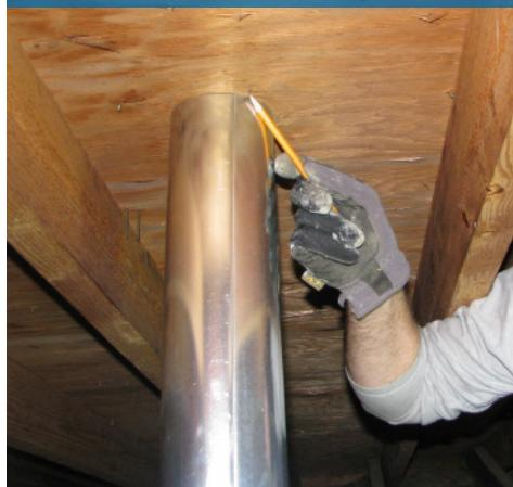
2. Drill small pilot holes along the edges of the traced template.
