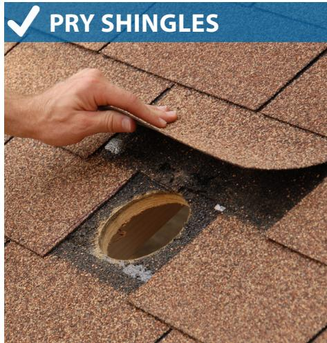
6. Install a steel flange vent cap under a row of shingles and directly over the hole, trimming shingles as necessary.
