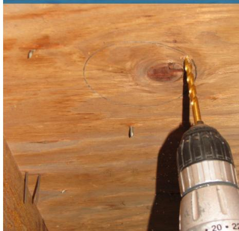
3. Outside of the house, trace the outline of the duct, using the pilot holes as a guide.
