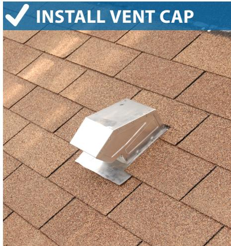
7. Seal the underside of the flange vent cap, nail holes and overlapping roof shingles with roof sealant.
