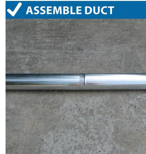
4. For the connection between the duct and the termination, install the duct adaptor supplied with the termination cap.
