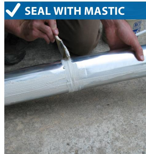
7. If installing a bath fan duct in unconditioned space, wrap the duct with insulation and seal the seams with mastic.
