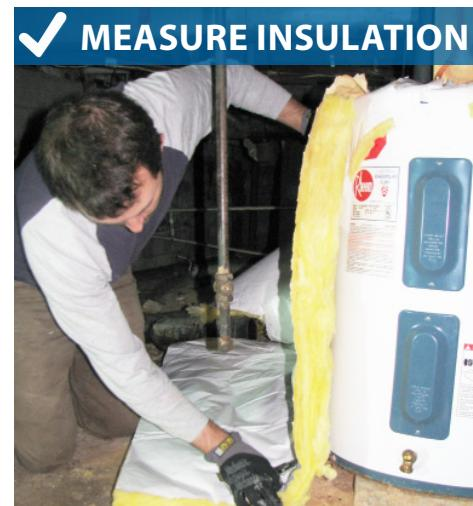
7. Cut a slit for the pressure-temperature relief valve and discharge pipe. Cut flaps for the electrical access panels.
