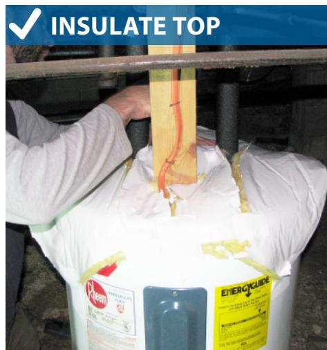
6. Cut insulation blanket to circumference of the heater. Position seam so it is not directly over the electrical access panels.
