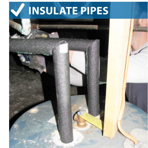
5. Cut a square piece of water heater insulation blanket for the top cutting slits for the pipes. Secure with tape without compressing the insulation.
