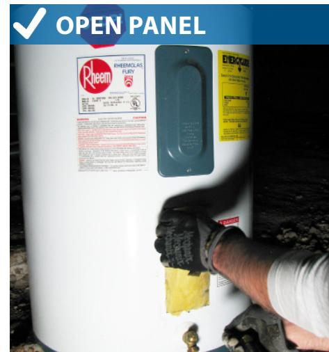
3. Use a screwdriver to turn all thermostats (if there are more than one) to 120 degrees Fahrenheit and close the electrical access panel.
