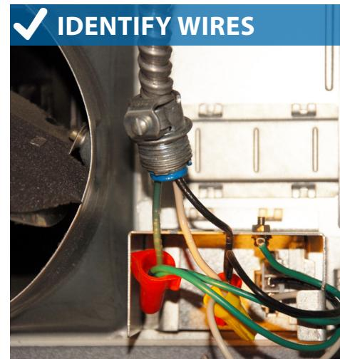
3. Disconnect the wires and remove from housing. Remove the fan and housing.
