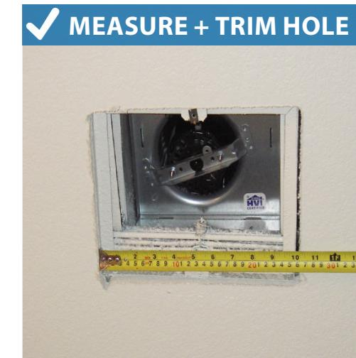
5. Install the new fan according to the manufacturer's instructions. Install the fan with the exhaust port aimed at the exterior termination.
