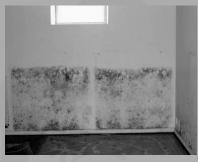
Basements and crawlspaces are often damp. The moldy walls in this picture are probably from rainwater that is not directed away from the house.
