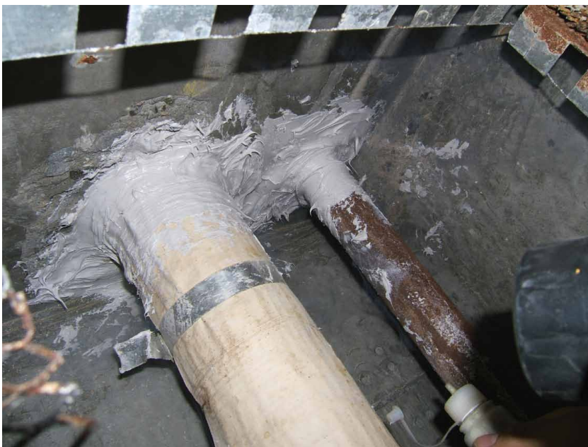
Figure 3 | Air sealing with fire stop around pipe penetrations between floors.
