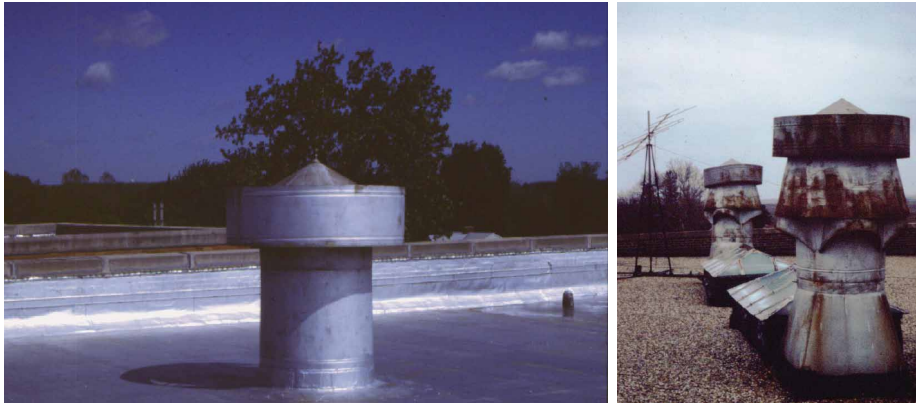
Figure 1 | Passive rooftop ventilators contain no fans. They depend on warm air rising and wind uplift to provide exhaust ventilation.
