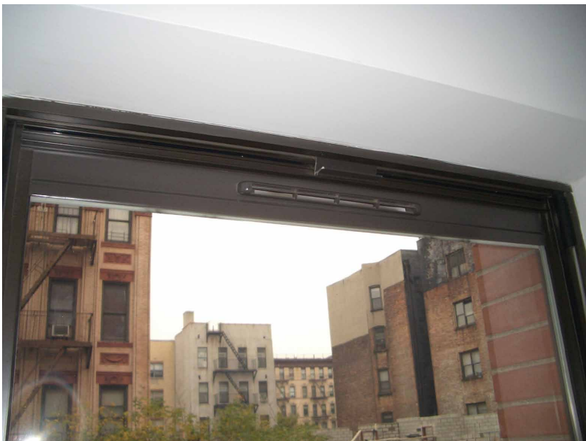
Figure 2 | Trickle vent installed in window frame.
