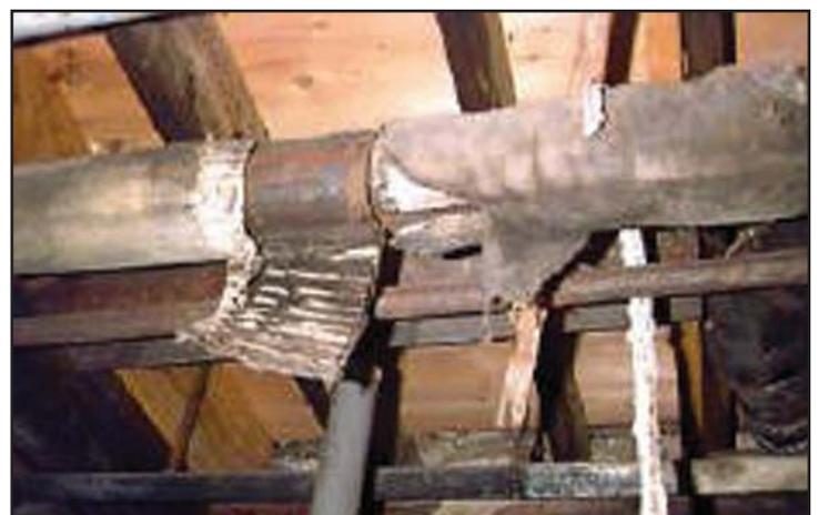
Figure 12.6. Heating Ducts Covered With Asbestos Insulation
