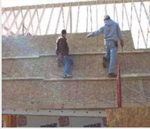
**L.** The subroof or roof sheathing is applied from the bottom up with temporary traction boards nailed to the subroof to allow safe installation of the material.
