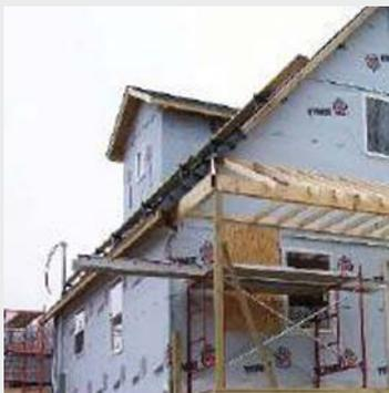
**N.** Flashing material, such as sheet metal, is installed at critical locations to make sure that water does not enter the home where the joints and angles of a roof meet:
