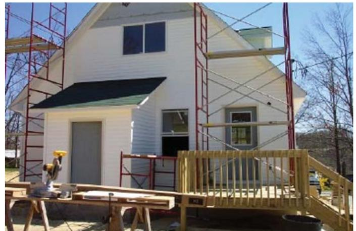
**O.** A safety scaffold is standing at the rear of the home, and the final roofing material has been applied, in addition to the exterior vinyl siding.
