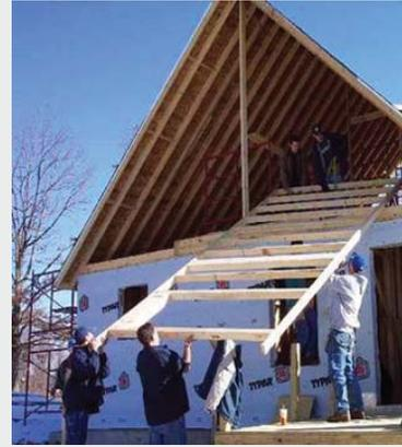
**M.** An interior wall is installed to create second-floor rooms.
